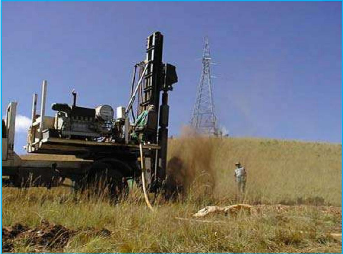
Figure 3-6: Foundations drilling
