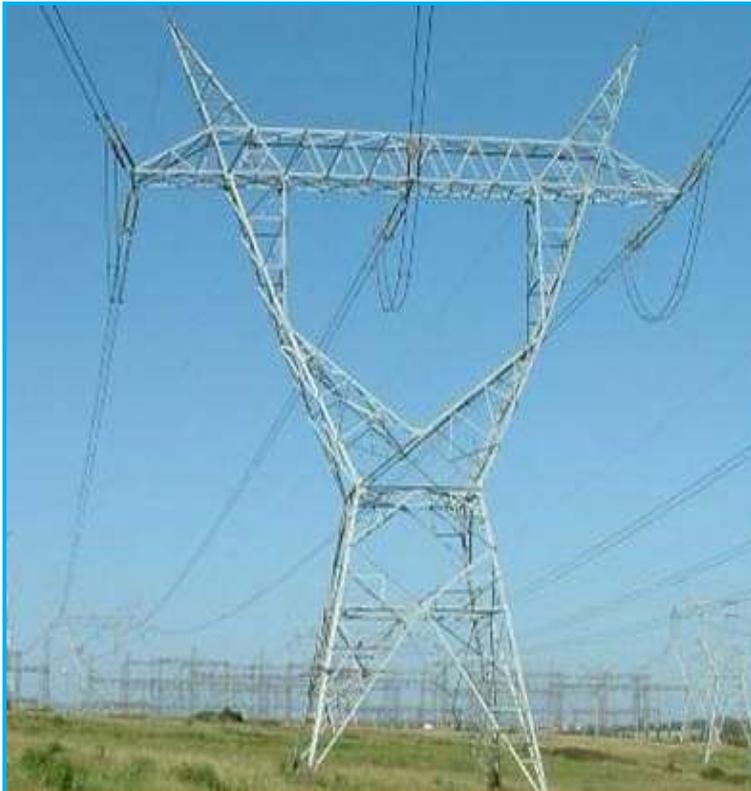
**Figure 4-1: Self-supporting Pylon**
